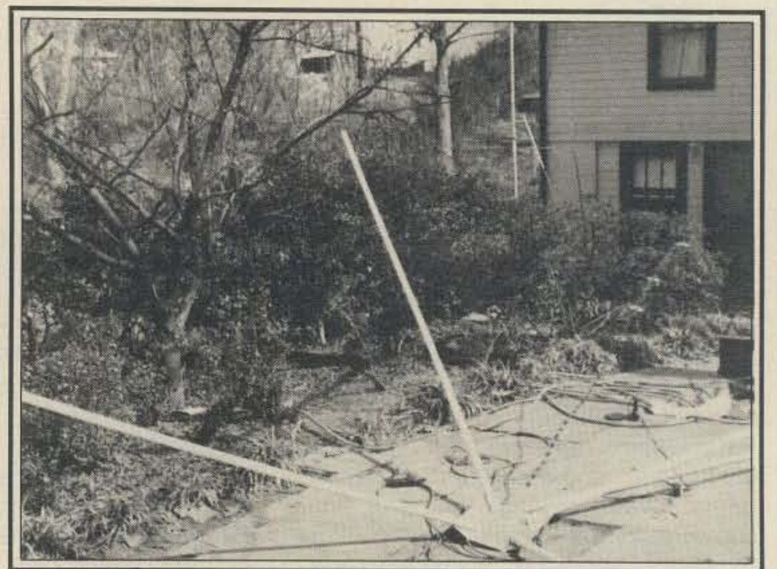
The reflector being assembled on the ground.
